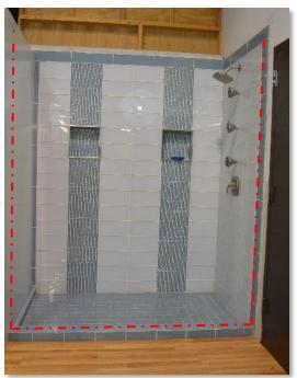
Determine the Centerlines of your unit. Note the fixed panel installs with the outside face of the glass 1-3/16" forward of the centerline (see illustration). The sliding panel should always be positioned closest to the shower head.
