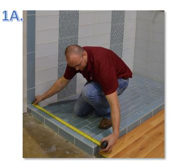
Measure and mark the center line of the Return Panel. Note the Return Panel goes 1-3/16" past the centerline of the Sliding and Fixed Panel. The forward edge of the Return Panel lines up with the outside edge of the Fixed Panel.
