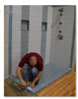
Install the Glass Clips in the proper position to match the notches in the glass.
