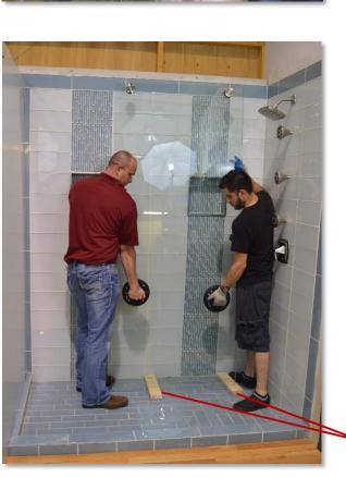
Lean the Sliding Panel against the back wall of the shower. Be sure the bottom edges of the panel are protected by wood blocks or cardboard.
