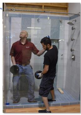
Position the Fixed Panel on the Centerline and with the Fixed Panel Retainers inserted into the holes.
