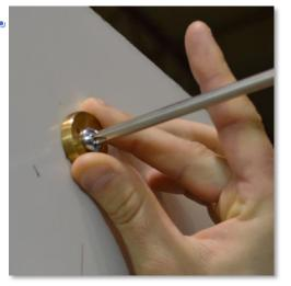
Using the screw and wall-plug provided, securely attach the Header Mount Bracket to the wall. Position the slot vertically and the screw in the center of the slot.
