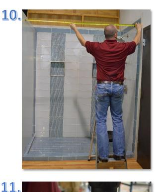
Measure the exact distance between the two blocks installed in Steps 3 & 4. Deduct  $\frac{1}{2}$ " and cut your header to the calculated length.
