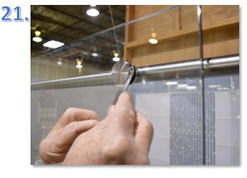
Attach the Fixed Panel to the Header with the Fixed Panel Retainers and usUse the wrench provided to securely tighten.
