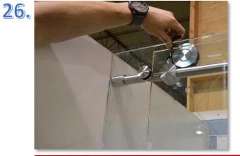
Adjust the remaining stop to set the open position of the door.
