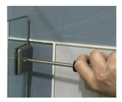
Install the Return Bracket thru the glass and tighten with the special tool available from Waterfall.
