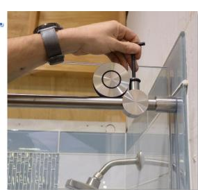
Adjust the stop to position the glass against the wall.
