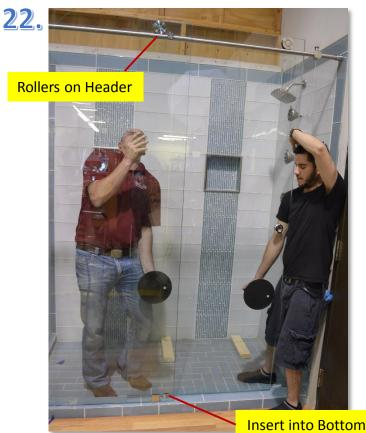
Lift the Sliding Panel into position with the Rollers resting on the Header and the bottom engaged in the Bottom Guide.
