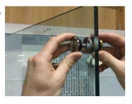
Install the Fixed Panel and securely tighten the Glass Clips
