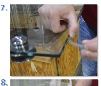
Use an Alcohol Pad to clean the edge of the Sliding Panel that meets the wall and install the Bulb Vinyl with the Double Stick Tape provided.
