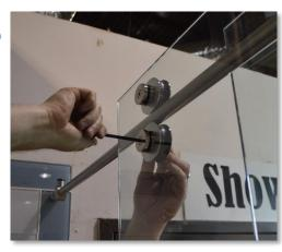
Install the Bottom Rollers and use the wrench to adjust to just barely contact the header,
