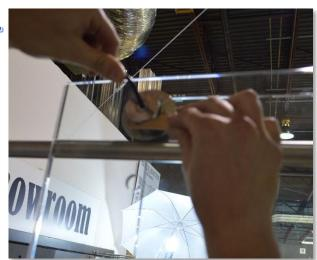
If the Sliding Panel is not parallel to the wall, loosen the roller screw and use the wrench provided to rotate the inner hub of the roller (reference Step 5). This rotation will raise and/or lower the top corner of the panel. After adjustment, securely tighten the roller screw.
