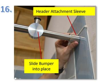
Before installing the header, slide the remaining bumper onto the header and loosely tighten.
