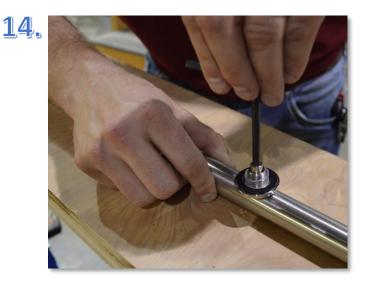
Install the Fixed Panel Glass Mount into the threaded hole away from the end of the header.
